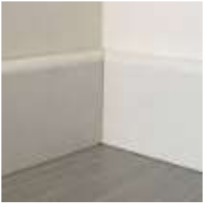
Skirting (excl. bathroom) 22x95mm Meranti Hardwood, to architects detail, painted
