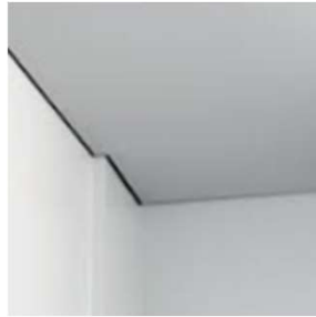
Cornices Shadow line cornice throughout
